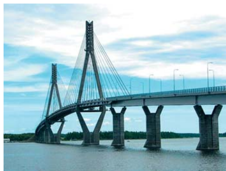
Most Replot – Raippaluoto, Finlandia
