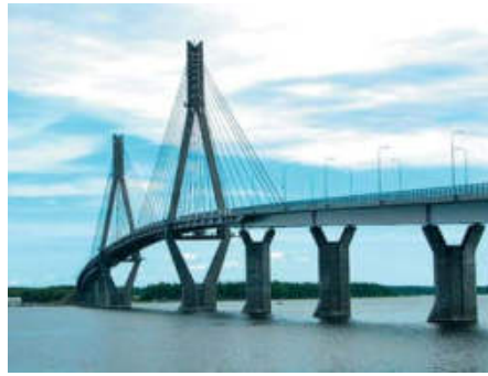
Most Replot – Raippaluoto, Finlandia
